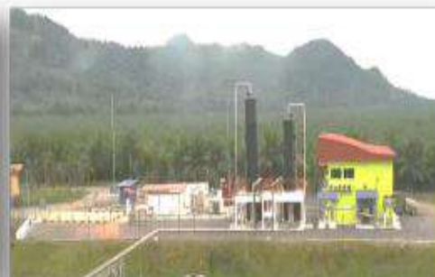
Biocompressed Natural Gas Plant Sg Teng 60,000 mmBTU/ annum
